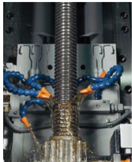
Conventional Too much quantity of oil is required.
