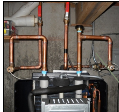
Heat Traps Correctly Installed
