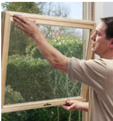
Install the upper sash
