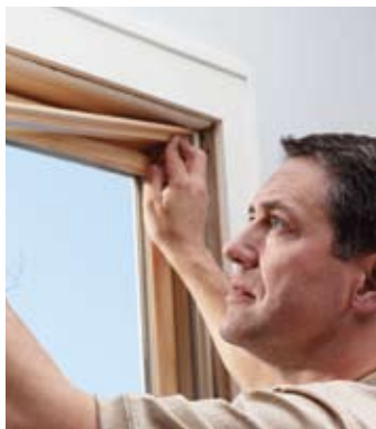
Install the wood head parting stop
