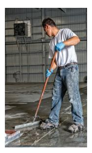
Once the condition of the floor and one environment are properly diagnosed and any mitigation steps taken, the next step is surface preparation. The surface of a concrete floor is prepared to increase the porosity, profile and surface area so that the new coating can penetrate, bond and effectively adhere to the concrete. Achieving a rough sandpaper-like profile is ideal. Surface preparation is always best accomplished with these three elements:
