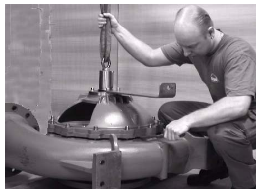
Fig. 2 Removing rotor unit
