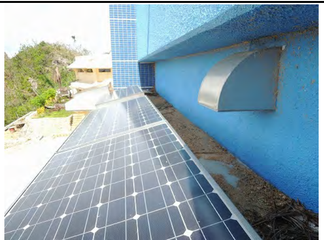
2F Eaves (Solar Panel Frame on the West Side)
