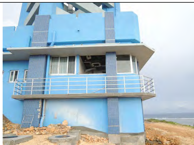
Observation Room from the South Side of the Facility
