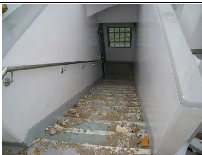
6F Radome Room (Staircase)
