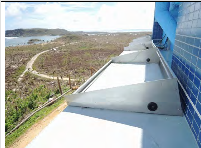
2F Eaves (Solar Panel Frame on the South Side)
