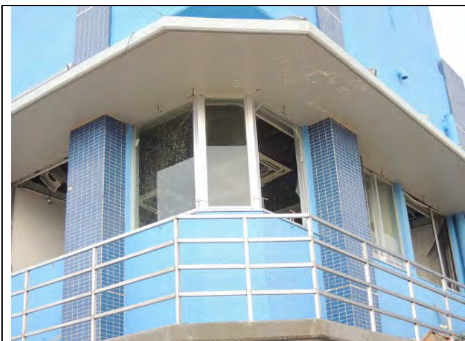
Observation Room from the Southeast Side of the Facility
