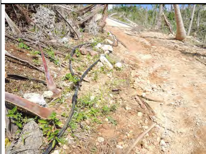
Water Supply Line of the Damaged Well
