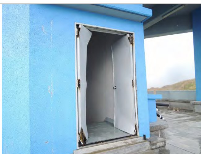
5F Observation Deck (Steel Door)
