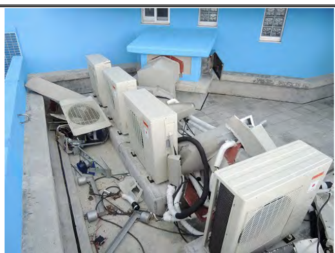
2F Roof (Air Conditioning Outdoor Unit Yard)
