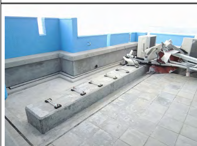
2F Roof (Air Conditioning Outdoor Unit Yard)
