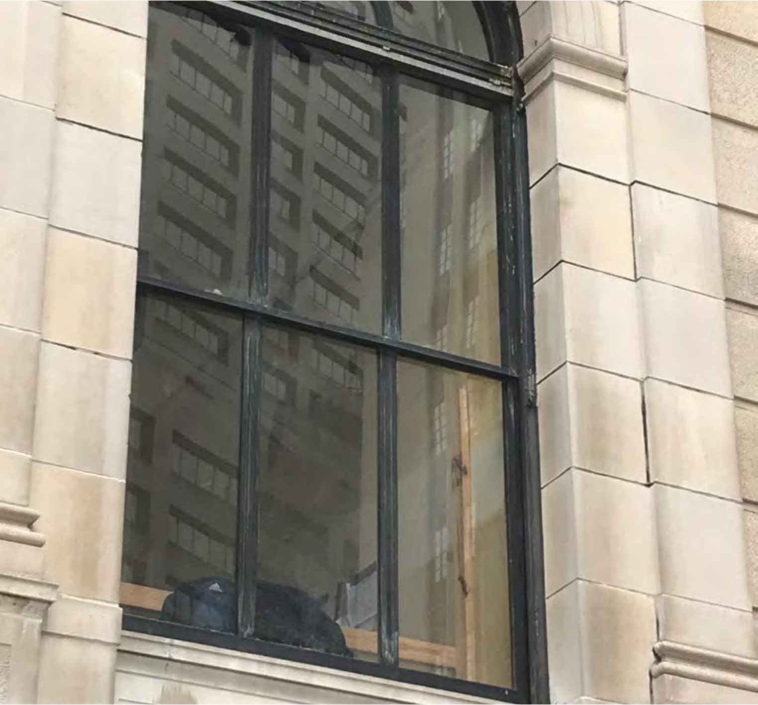
LEVEL 2 TEST WINDOW FOR DOWSIL SEALANT & SEALANT TAPE (RIGHT)
