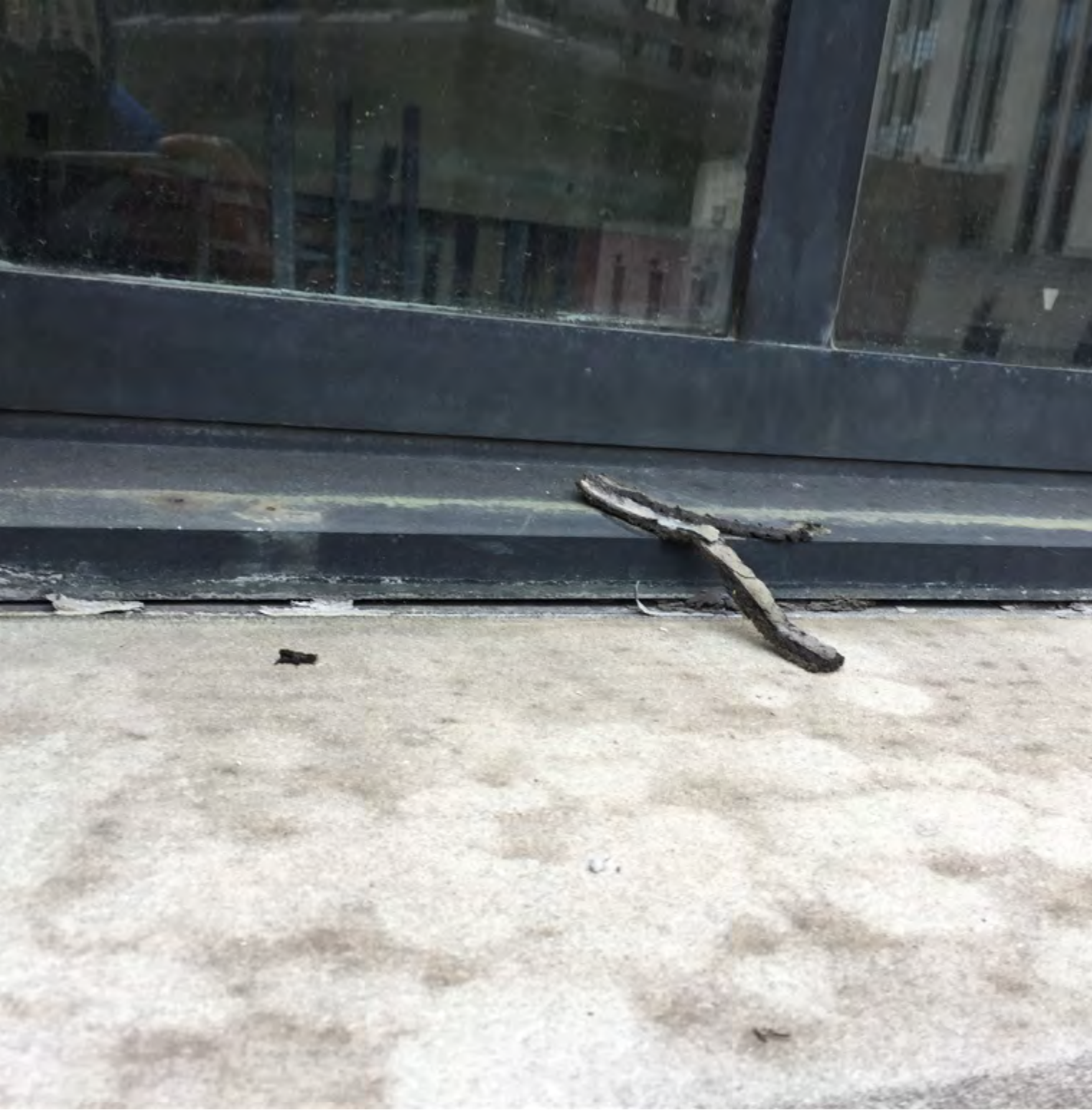
EXISTING FAILED SEALANT: INTERIOR DETERIORATION AS OF 12/04/19
