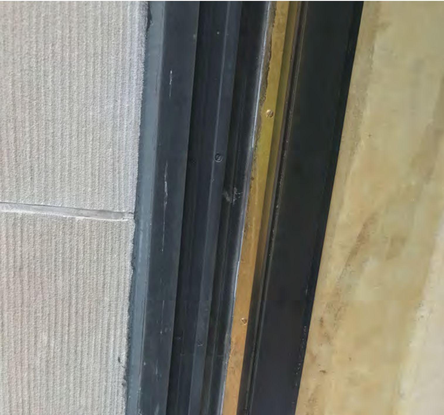
CLOSEUP VIEW OF DOWSIL SEALANT 790/791/795 (LEFT JAMB)
