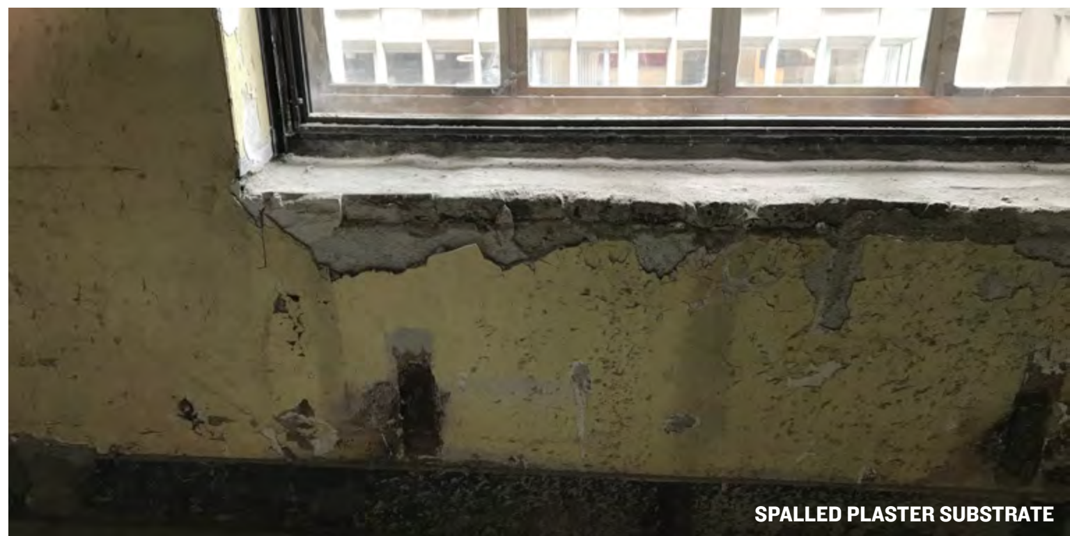
FAILED PLASTER FINISH
