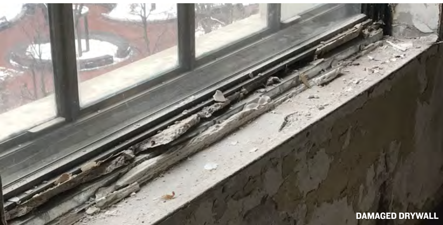
DAMAGED WOOD SILL BLOCKING
