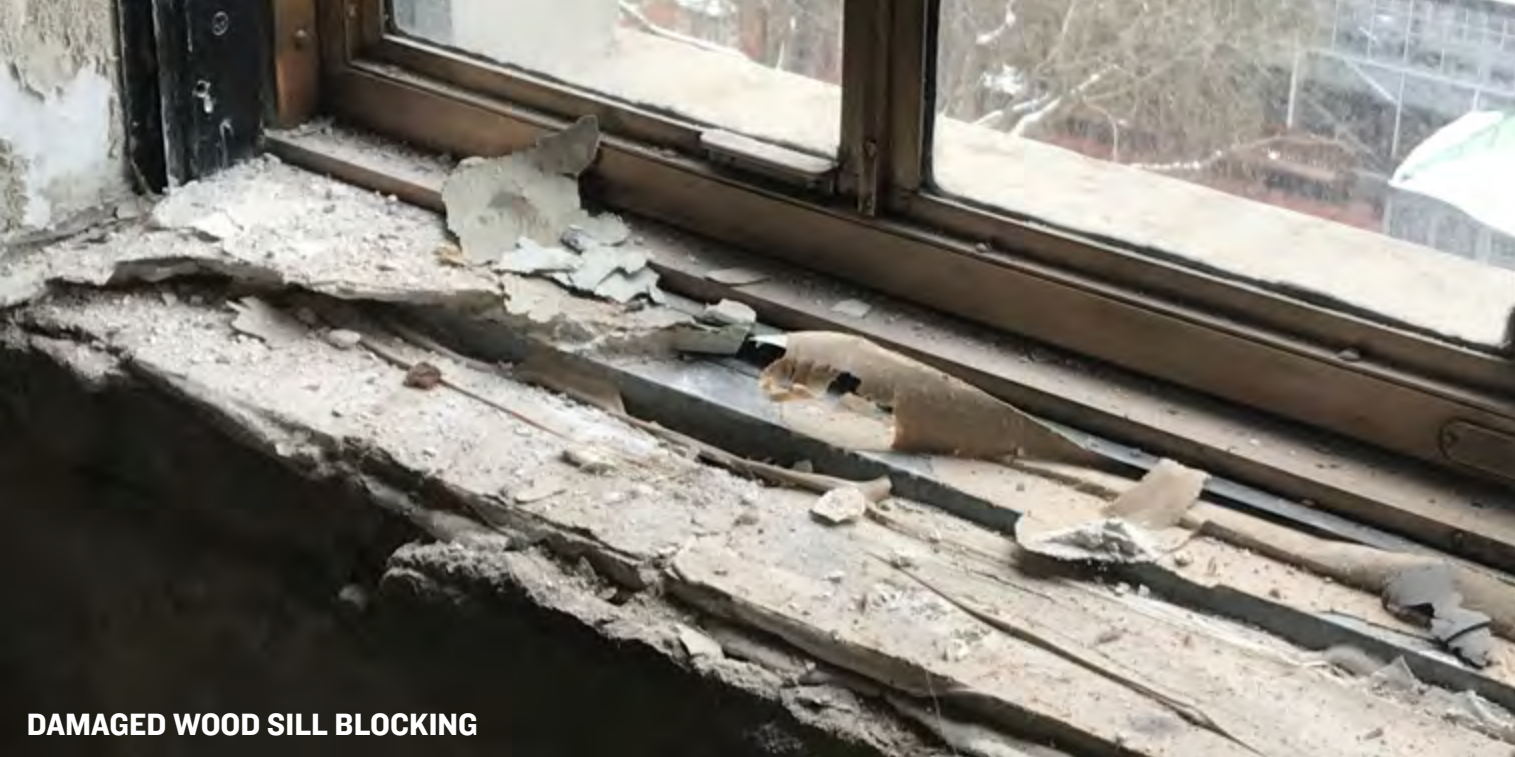
FAILED PLASTER FINISH
