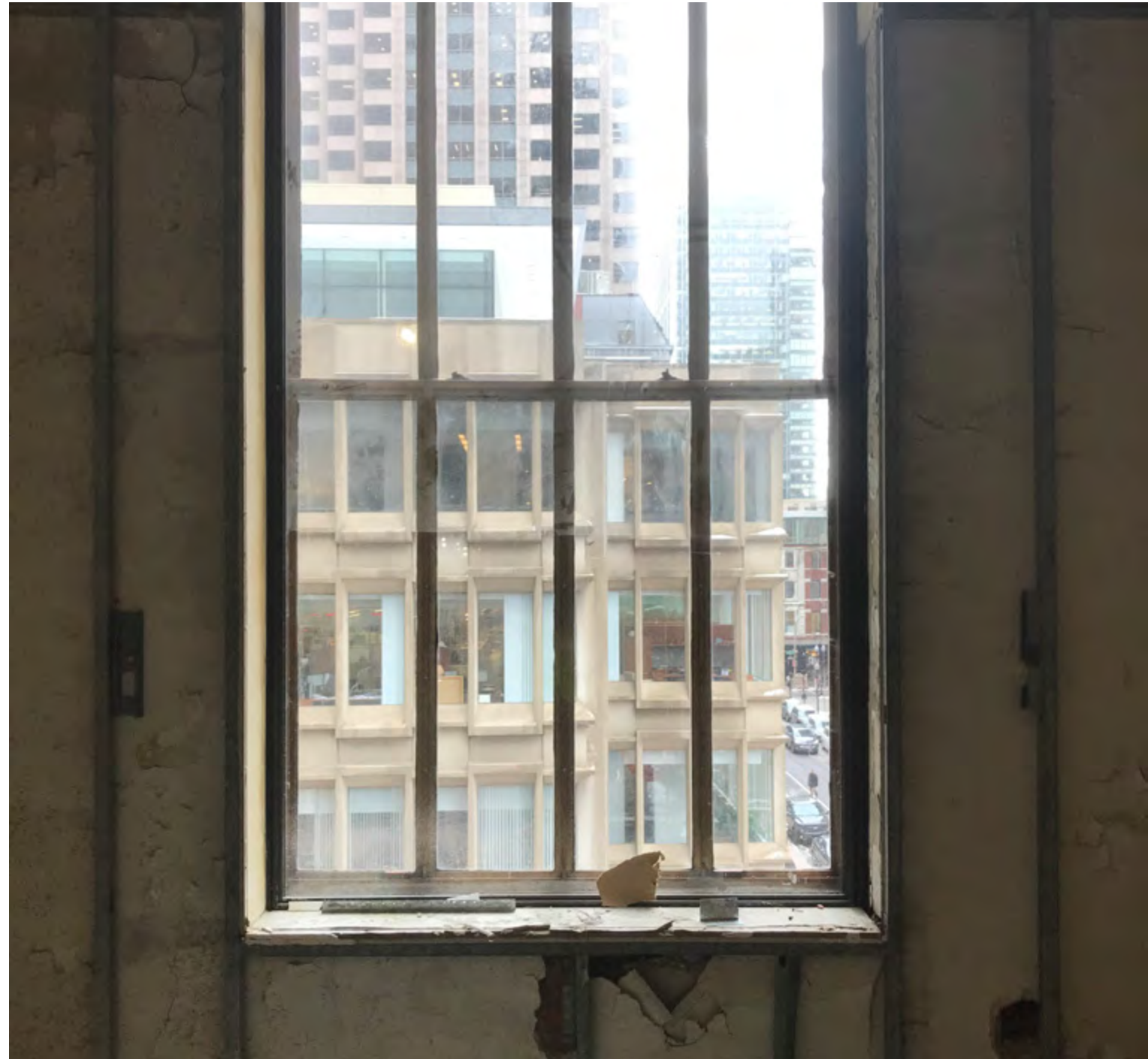
STUDS TO RECEIVE ROCKWOOL INSULATION AND DRYWALL
