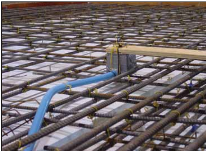
Figure 4.1.n. Blockout of foam around edge handling insert.
