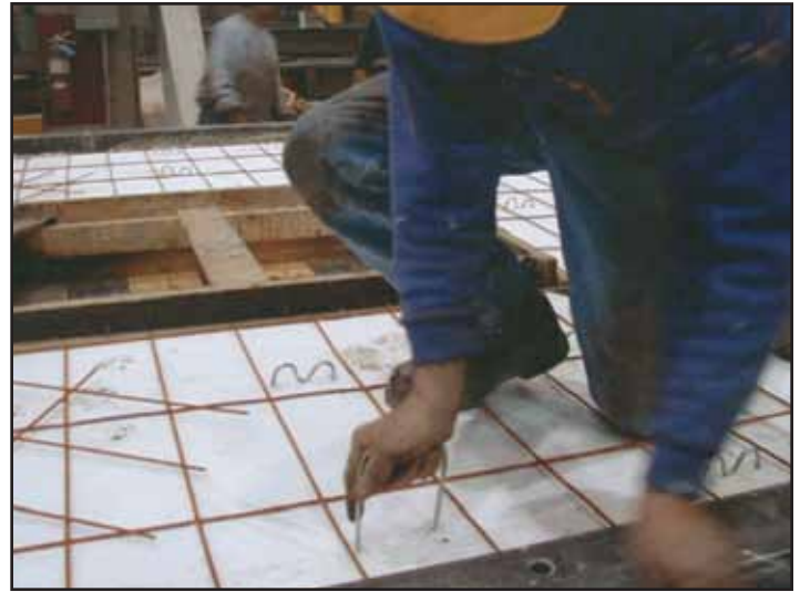
Figure 4.1.j. Stainless steel pin connectors for connecting wythes.
