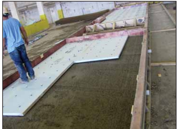
Figure 4.1.f. Insulation partially in place.
