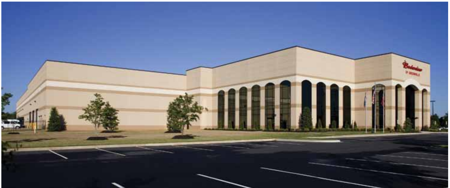
Figure 1.5.q. Budweiser Warehouse, Roebuck, S.C.
