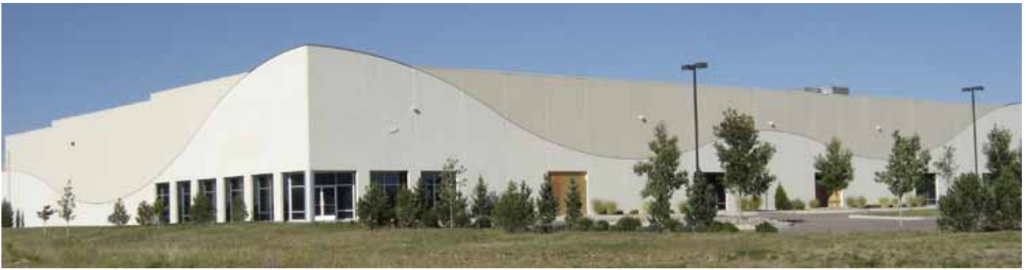
Figure 1.5.w. Aero Tech Warehouse, Colorado Springs, Colo.
