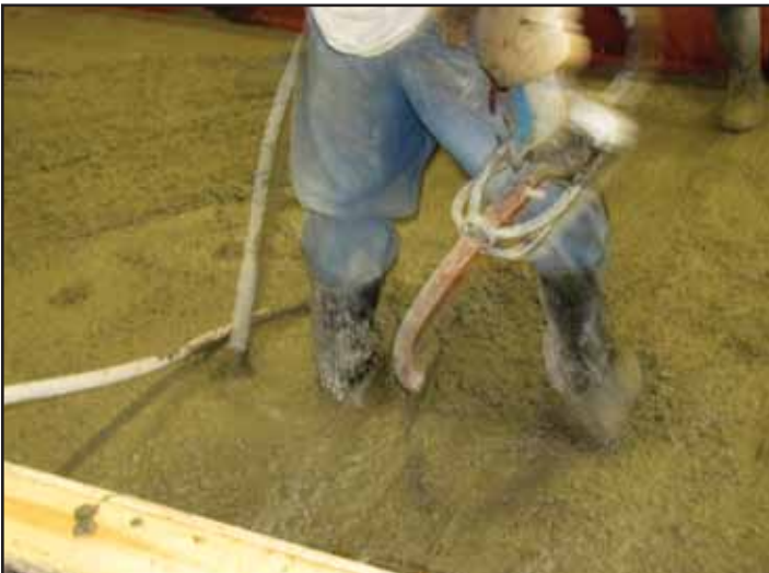
Figure 4.1.c. Vibrating face mixture using internal vibrator.
