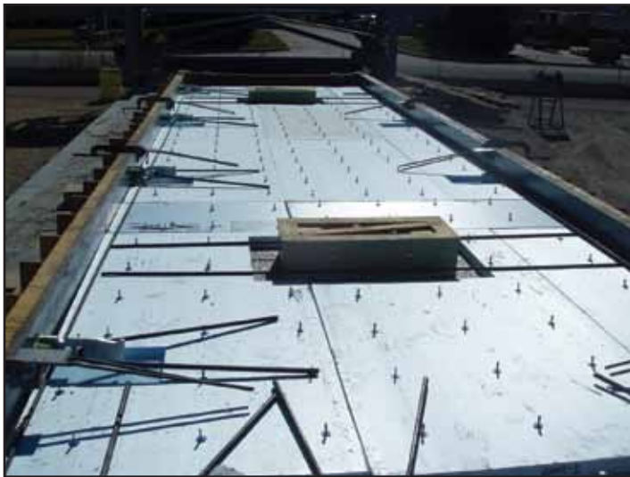
Figure 4.1.m. Electrical conduit and outlet box in place.
