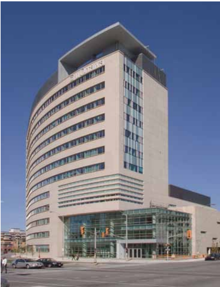
Figure 1.5.d. Desmarais Building, University of Ottawa, Ottawa, Ontario, Canada.
