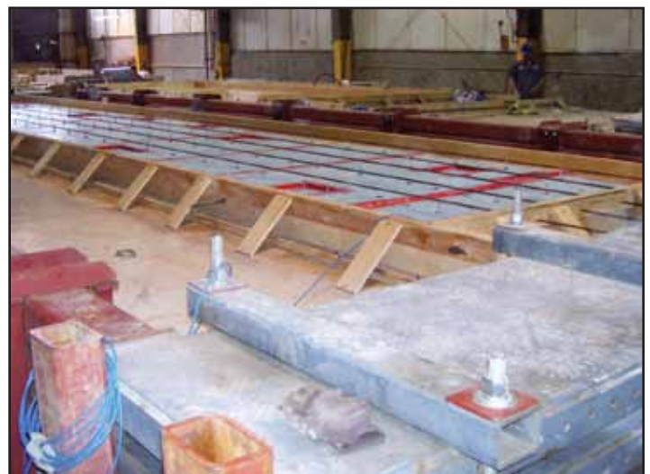
Figure 4.1.l. Prestressing strand in place to prestress panel.
