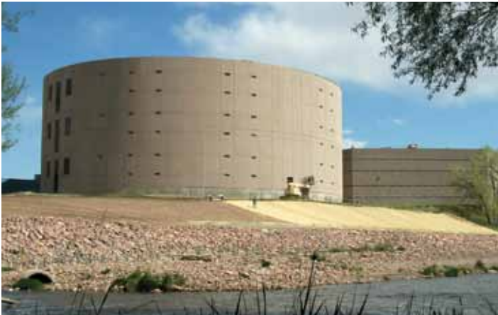
Figure 1.5.x. El Paso County Correctional Facility, Colorado Springs, Colo.
