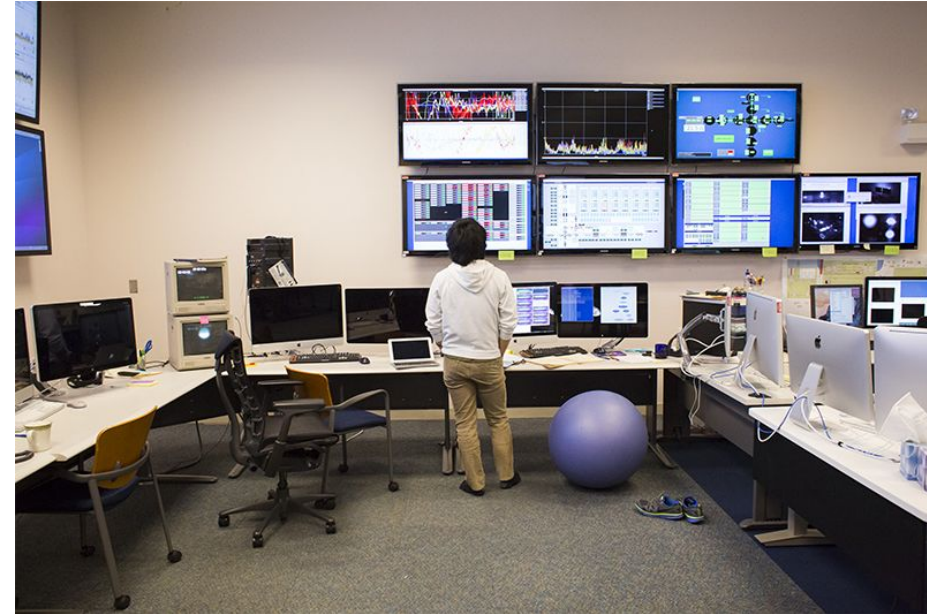
LIGO control room
