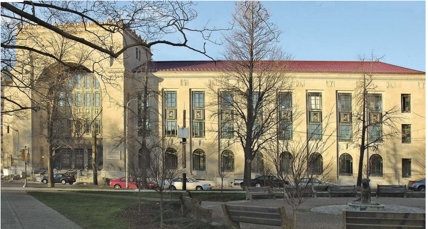
Perelman Building 2501 Fairmount Avenue
