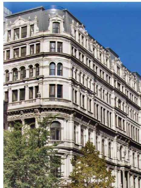
The Victory Building 1001-13 Chestnut Street
