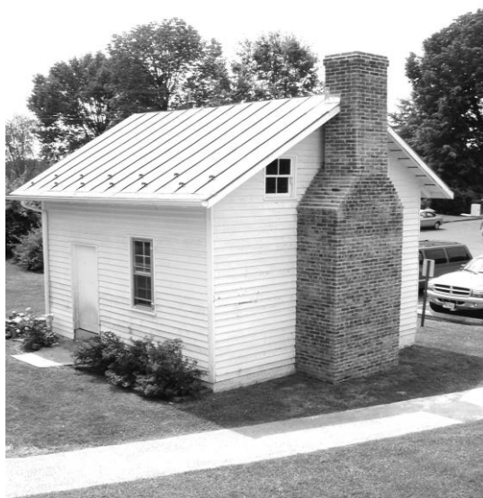
Law Office with new chimney
