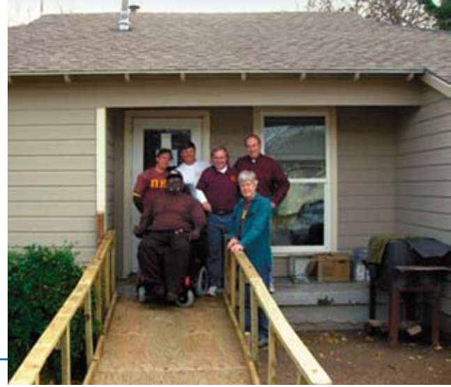
A finished ramp brings smiles to all.
