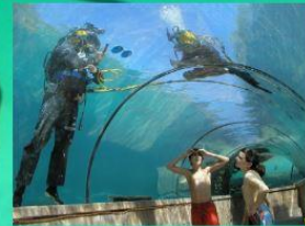
Leak Detection and Repair
