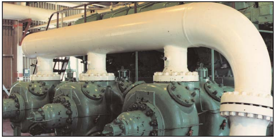
Pulsation Bottles, Extruded per ANSI B31.8 (as shown) or fabricated and stamped to Sec. VIII.
