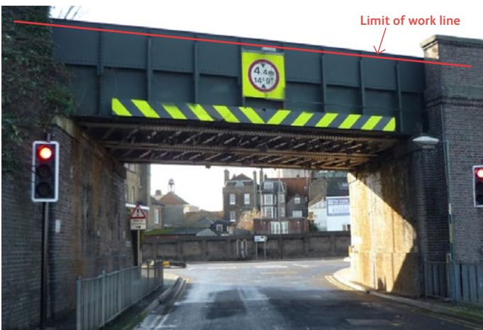
Figure D4: Solid parapet bridge
