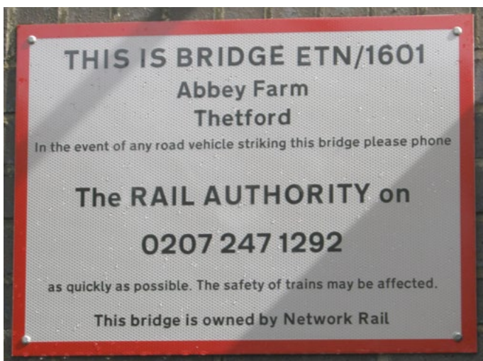
Figure 4: Network Rail bridge identification plate
