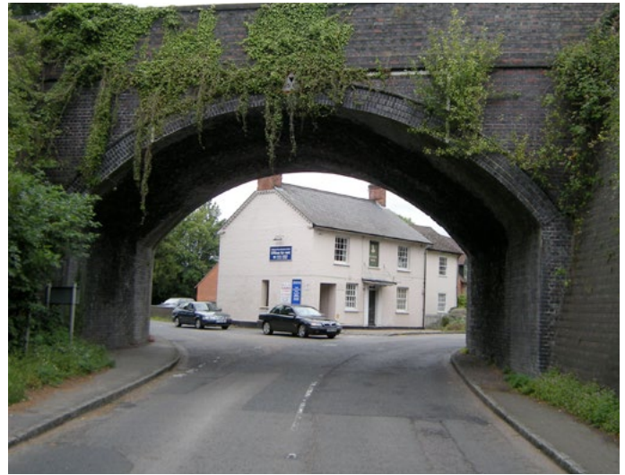
Figure D3: Vegetation on the bridge elevation obscuring the traffic sign
