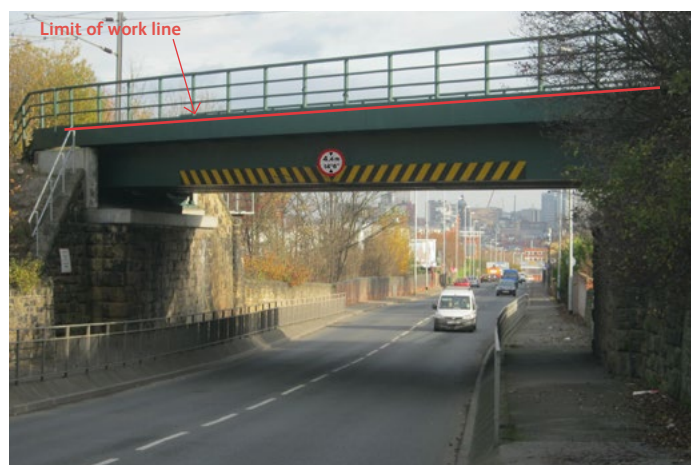
Figure D5 - Open parapet bridge
