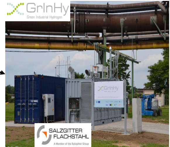
150/30kW Reversible electrolyzer at Salzgitter, Germany High-temperature Electrolyzer as reversible generator (rSOC, reversible Solid Oxide Cell, to produce either hydrogen or electricity) in the industrial environment of an integrated iron/steel plant (exploiting also high temperature heat available)
