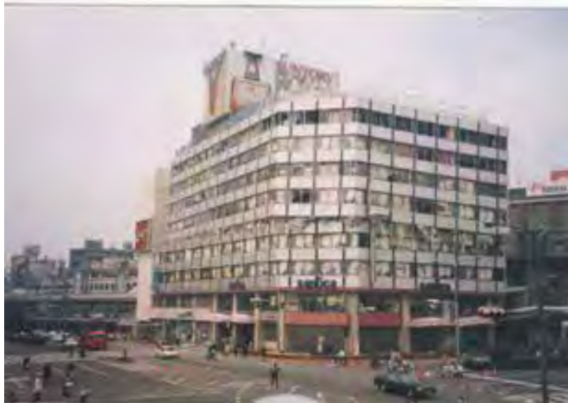
Fig. 5. Heavy damaged office building with torsionally flexible system during the earthquake in Kobe 1995
