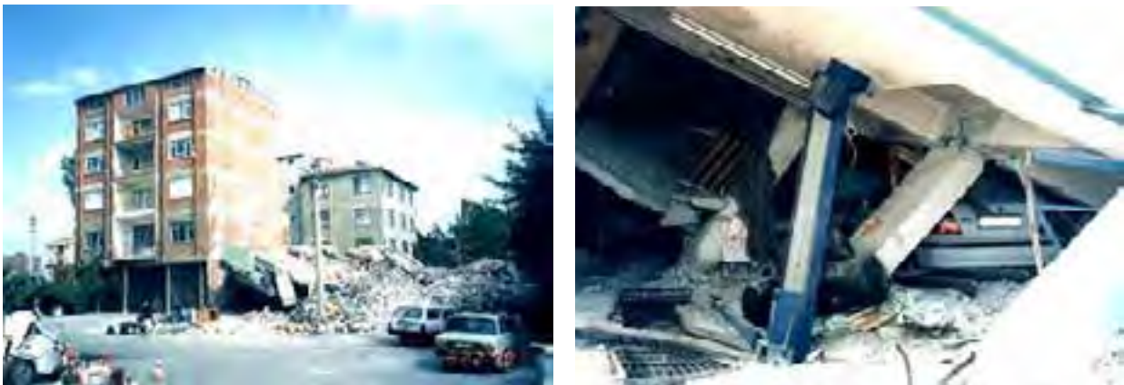
Fig. 28. Total collapse of a building due to “weak columns-strong beams” – Turkey 1999
