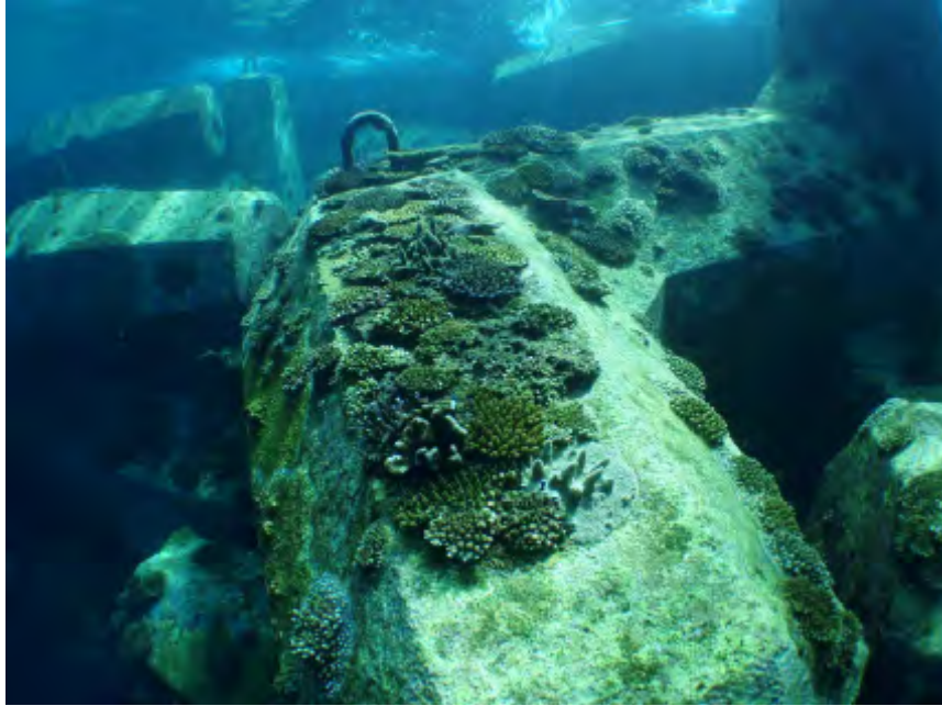
Figure 1: Corals covered on the wave-dissipating “Eco-Blocks” at Naha Port, Okinawa. The “Eco-Blocks” were placed 8 years ago. The photo was taken in August 2007. (Courtesy of Okinawa General Bureau).
