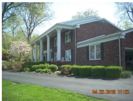
Figure (1) Exterior Picture of house.
