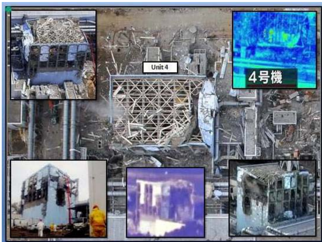
Figure 6: Damage to Unit 4
