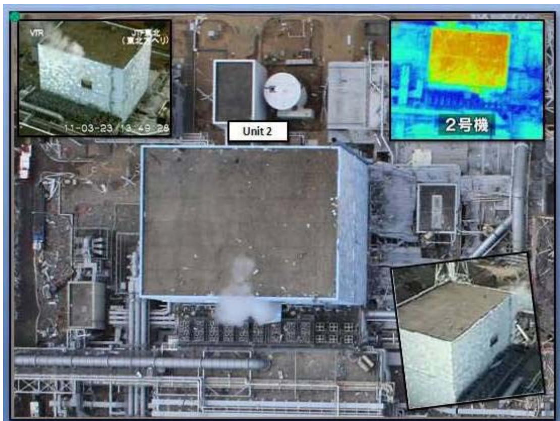
Figure 4: Damage to Unit 2
