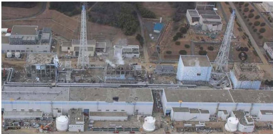
Figure 7: Fukushima Dai-ichi Units 1-4 following explosions
