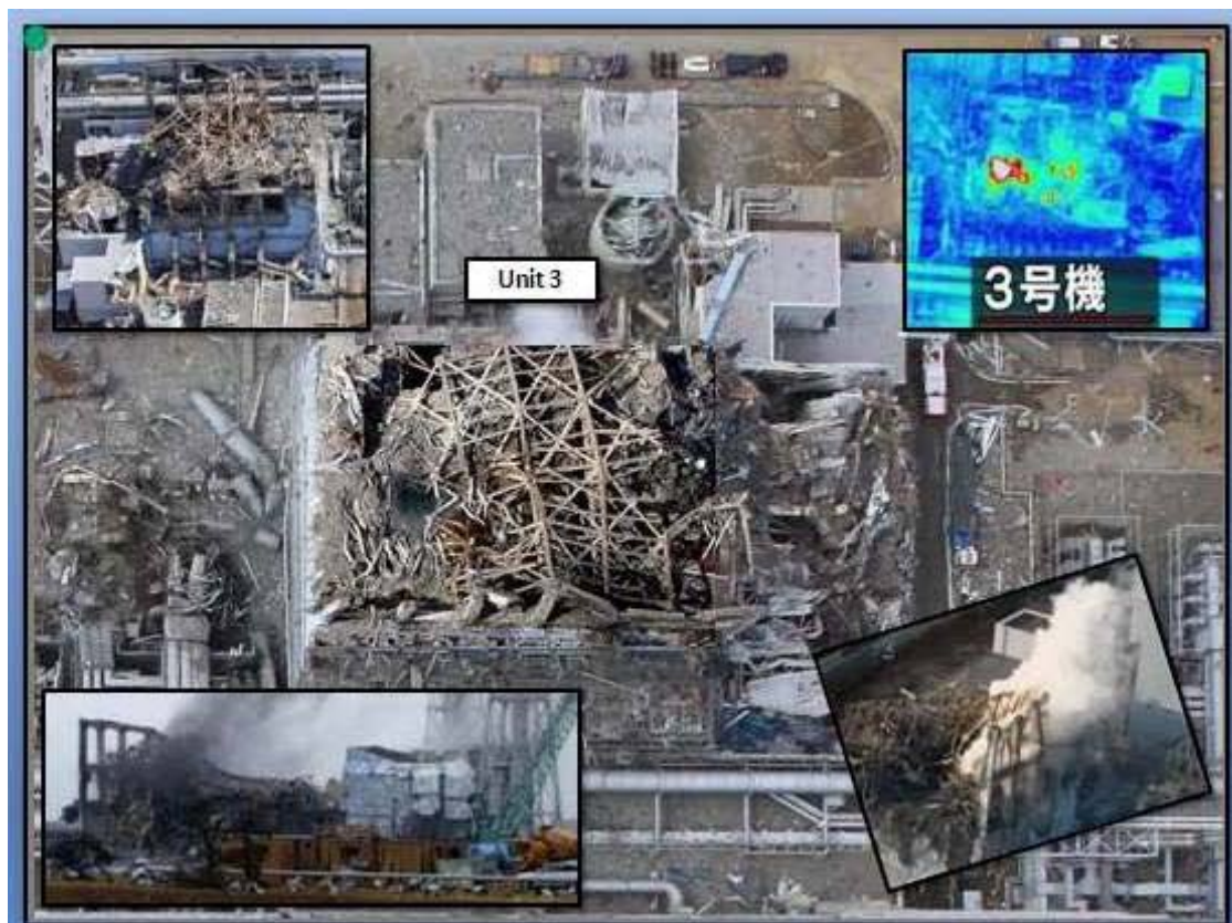
Figure 5: Damage to Unit
