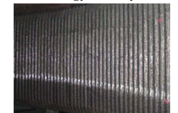
Overlay welding is used to weld Inconel alloys to heat exchangers
