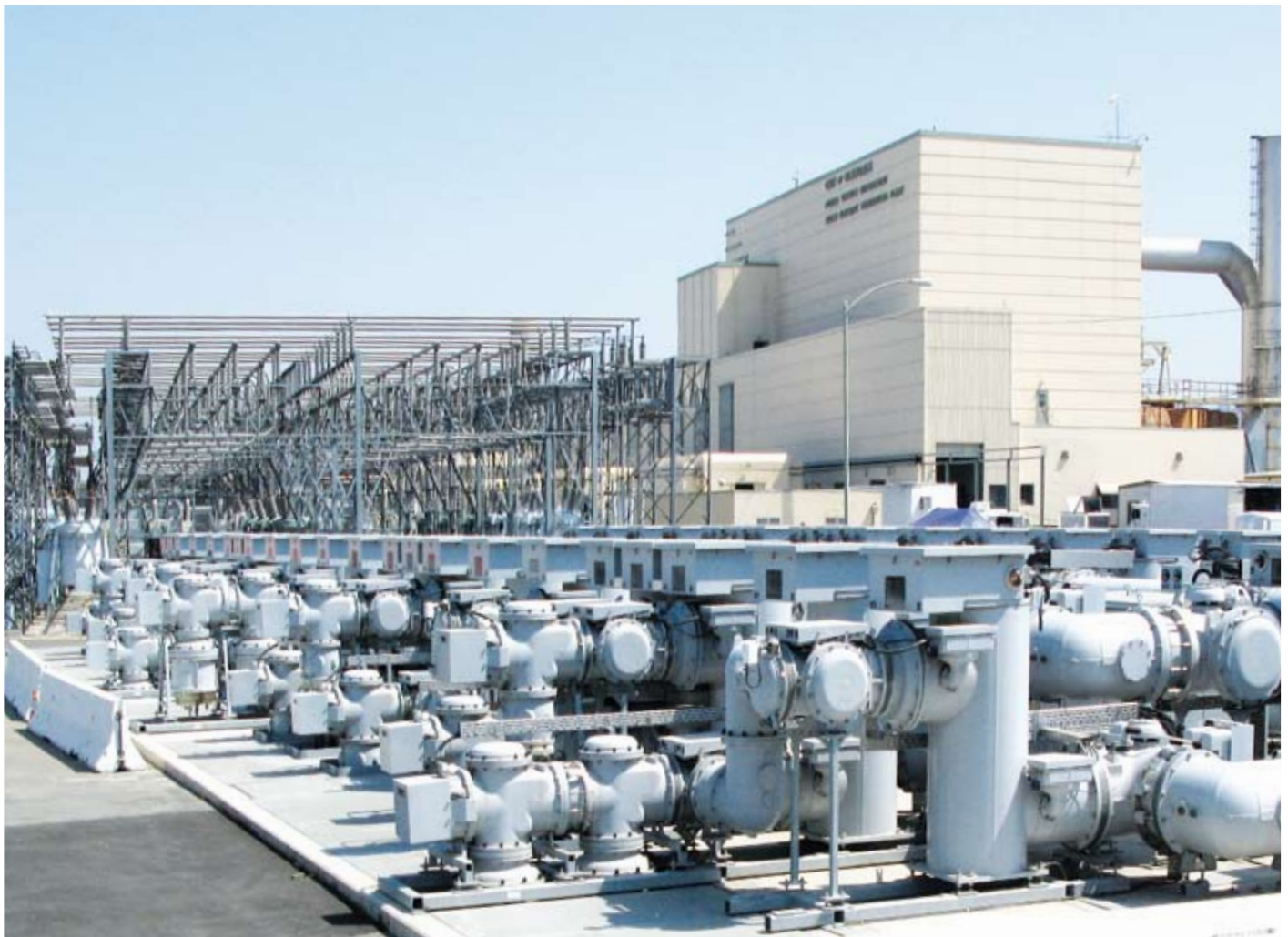
ELK-04 in 1½-circuit breaker arrangement, outdoor installation in front of a conventional air-insulated switchgear
