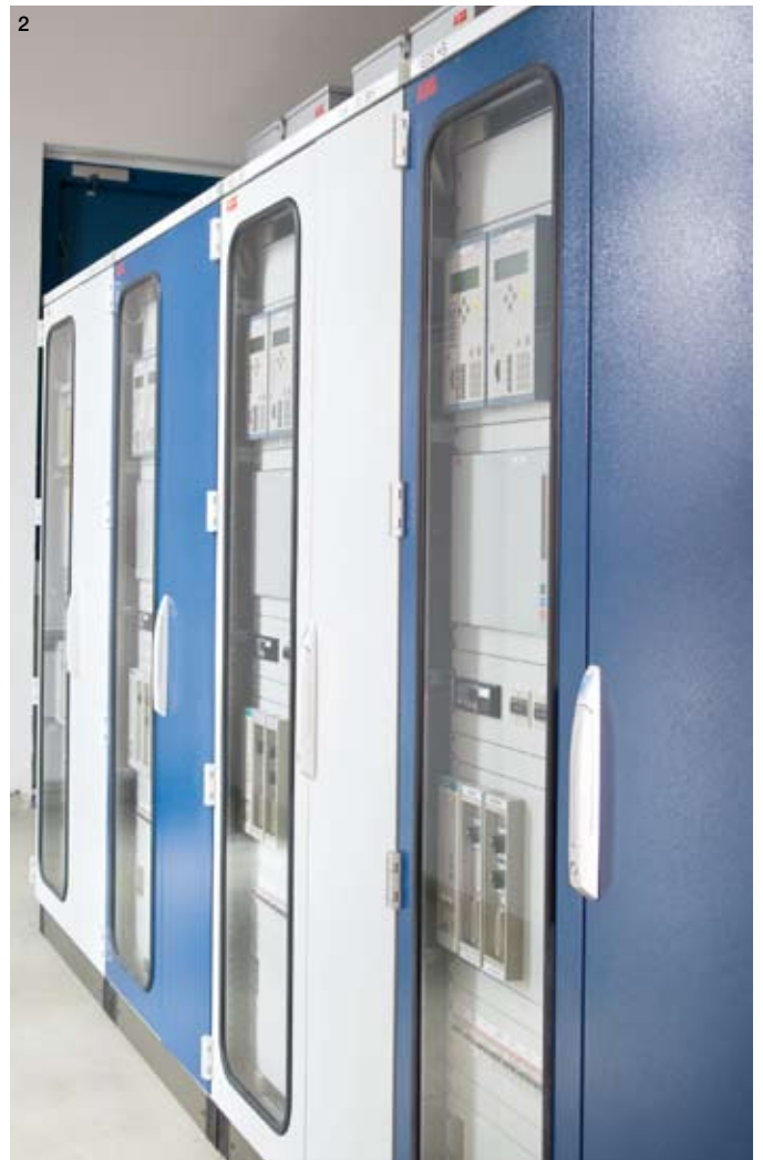
1 Human-machine interface of digital control device | 2 Local control cabinets with digital control and protection
