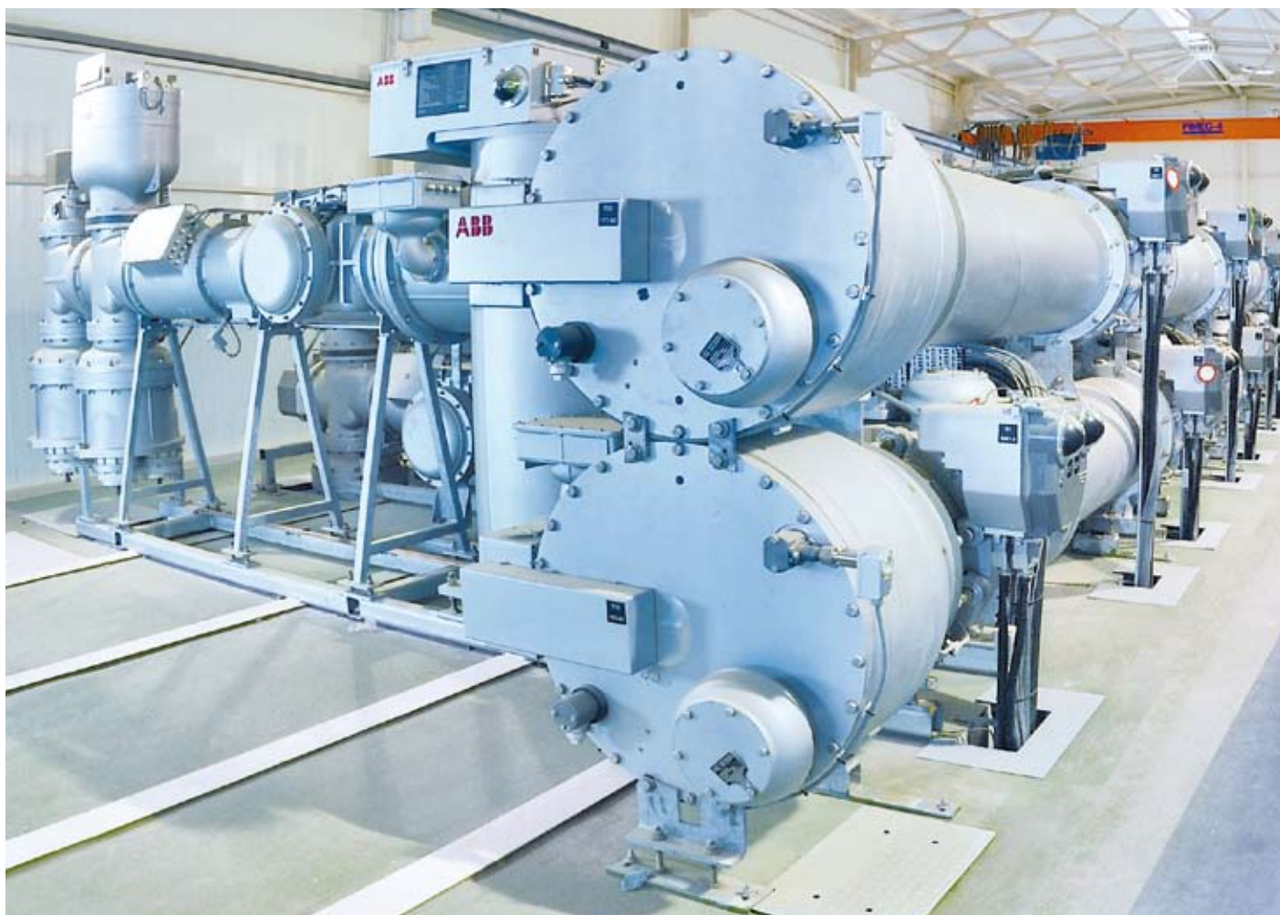
ELK-04 in 1½ circuit breaker arrangement
