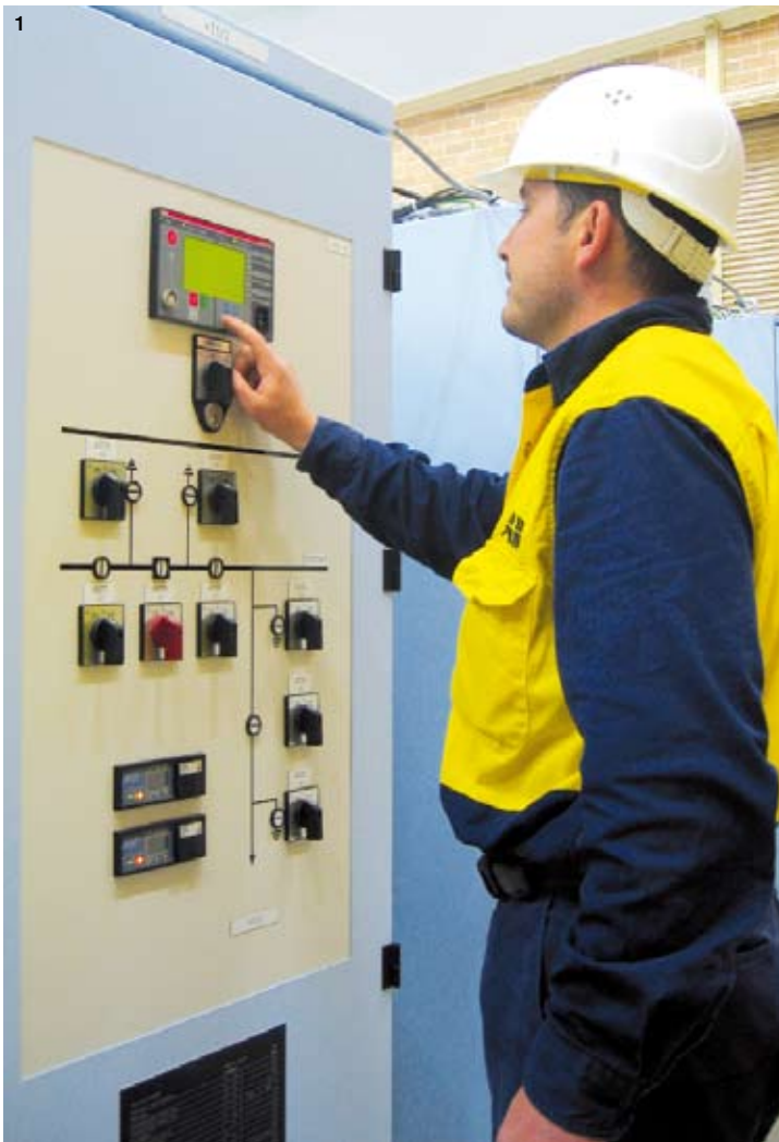
1 Human-machine interface of digital control device | 2 Local control cabinets with digital control and protection
