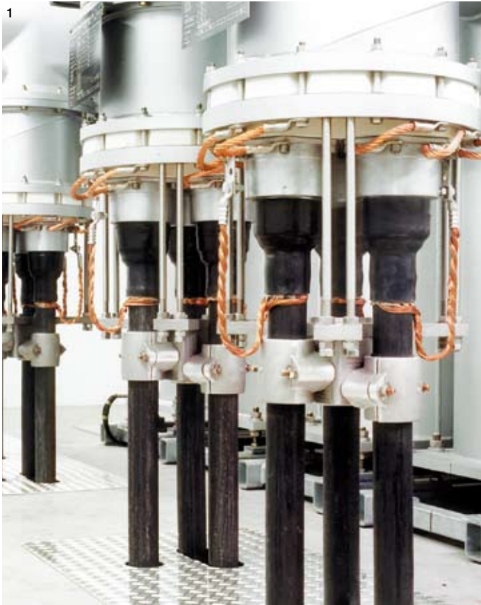
1 Plug-in dry type cable connection | 2 SF 6 -Gas-to-air bushing to connect overhead lines
