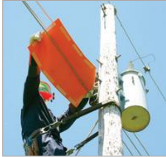
Installing a Zip-On Blanket
