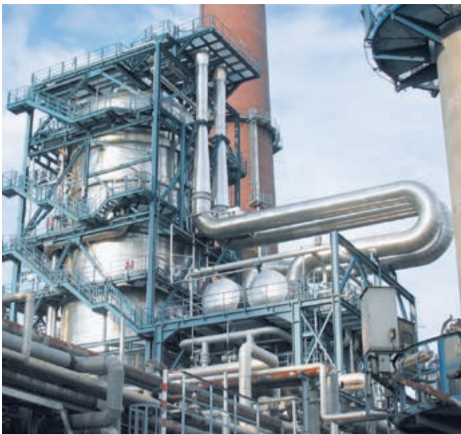
Fig. 4 3-stage steam jet vacuum pump with surface condenser for the vacuum column of a refinery Suction flow: 13 180 kg/h (436 000 m 3 /h) Suction pressure abs.: 4.5 kPa abs. Discharge pressure abs.: 110 kPa abs.
