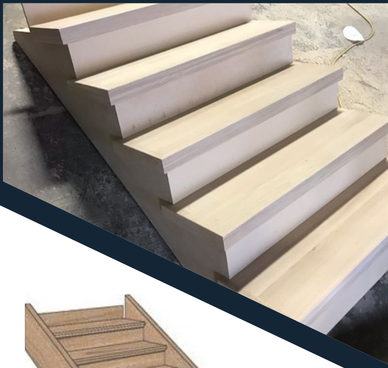
Closed Risers with Closed Stringer
