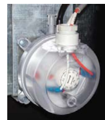
Clogged Filter Alarm
