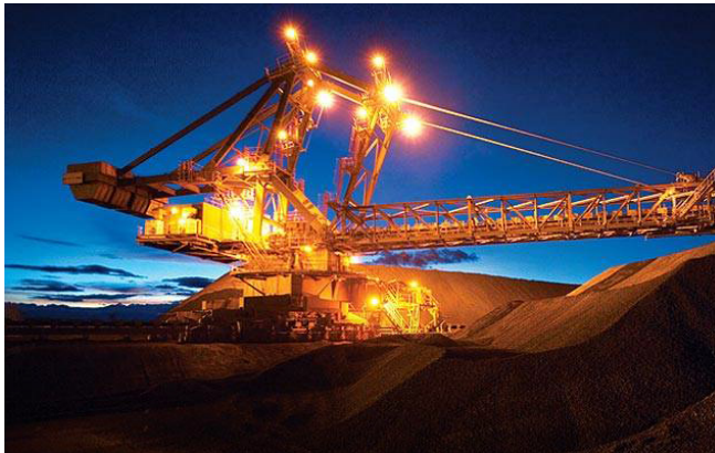
AREA C IRON ORE MINE, WESTERN AUSTRALIA, LEIGHTON CONTRACTORS © Leighton Holdings leighton@leighton.com.au
