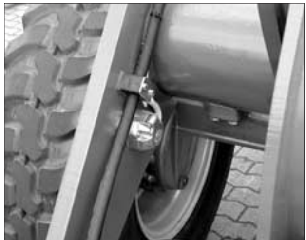
Front Electrical Socket
