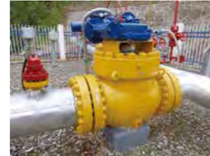
Puguang project in Sichuan, China
