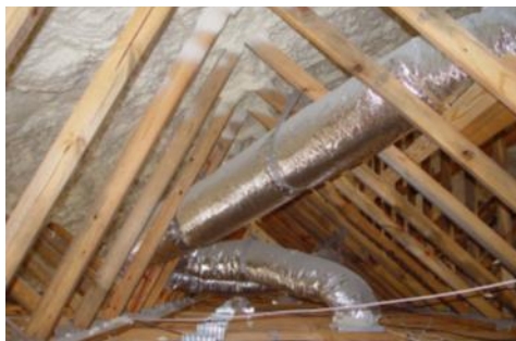
Figure 7: SPF Insulation Installation
