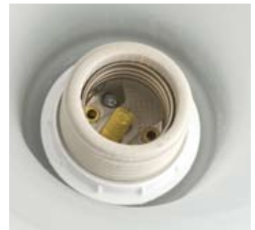
Shade secured in place.
