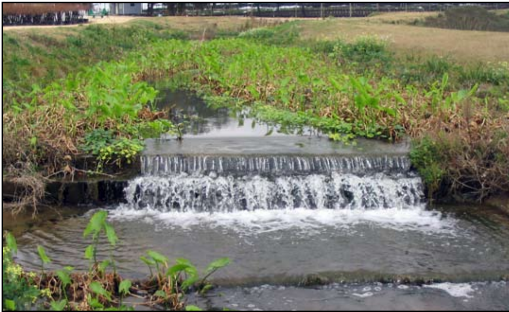
Figure 4. Nitrification structures (elevation changes where runoff is aerated) enhance conversion of ammonia to nitrate, the nitrogen form removed in constructed wetlands.
