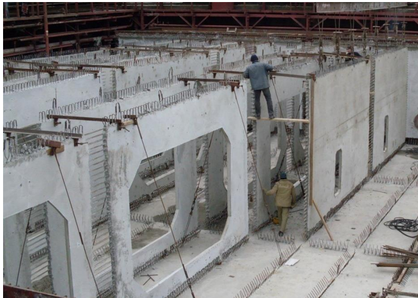
Figure 1: Construction technology of concrete floating structures at the Kherson State Plant "Palada" (Kherson, Ukraine).
