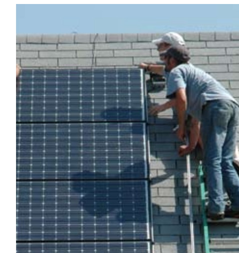
Installers position the WISE program's PV array.
