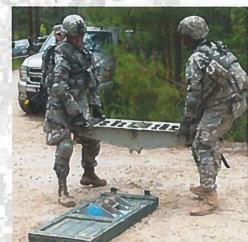
Task: Two Soldier Task; Assist in the Construction of a Bailey Bridge
