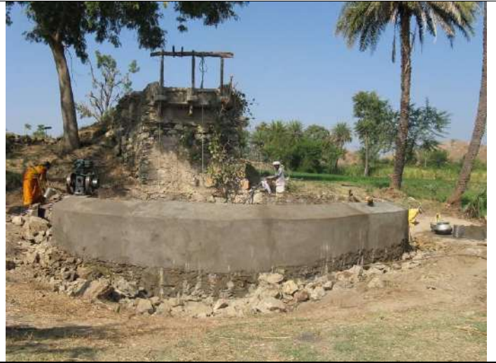
Newly developed well boundary/lining at Sawna village
