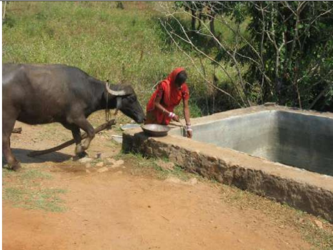
A 21,000 l water tank satisfying community need
