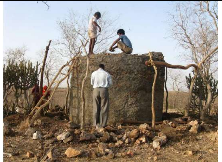
Water tank under construction in Vasatalab
