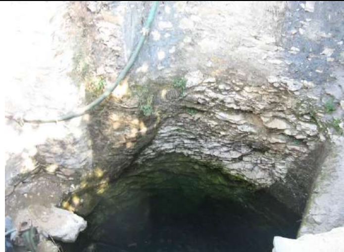
Water quality improved due to well lining at Alukheda
