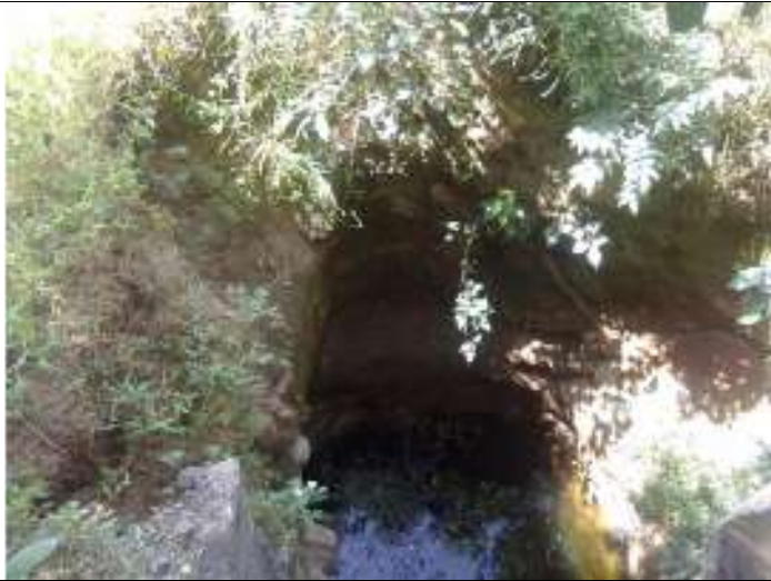
Boundaryless well in Alukheda – before well lining. Mud flows easily in the well.
