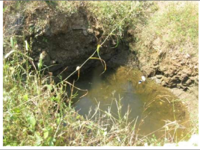
Water pollution due to absence of boundary around the well in Ramela
