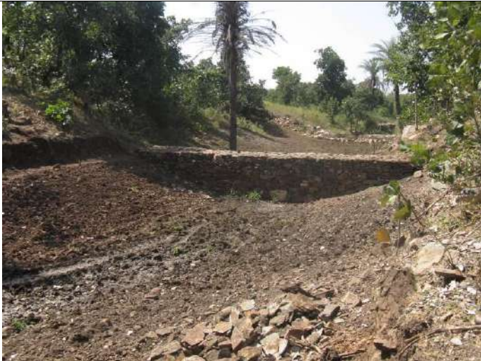
LSCD build across the stream in Alukheda
