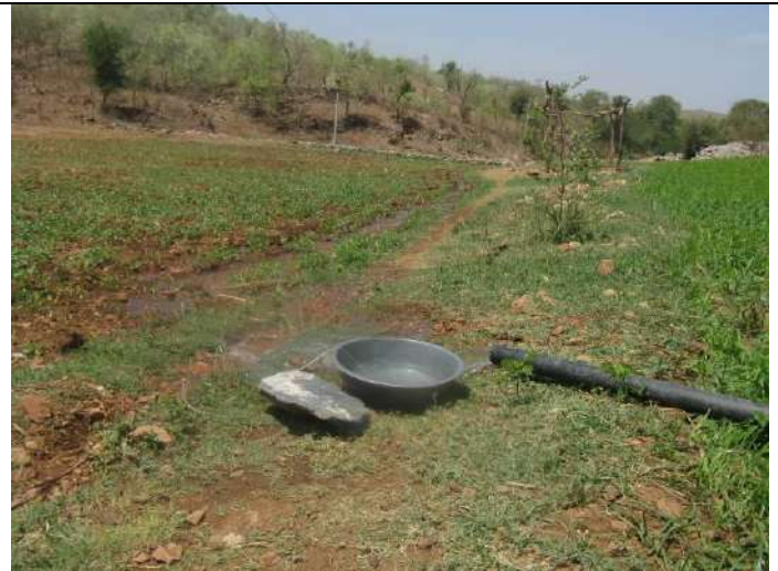
Pipeline under use in Moklatalab. Extra land irrigated from pipeline
