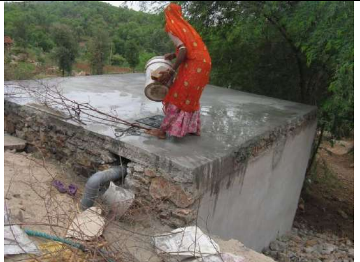
A community women at Hathida watering the RRWHS surface for fixing cement
