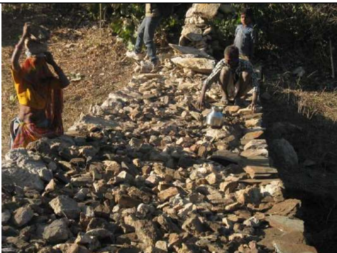
LSCD under construction on individual farm
