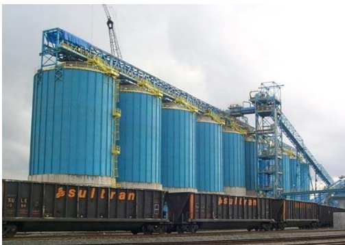
Completed battery of 48' diameter silos
