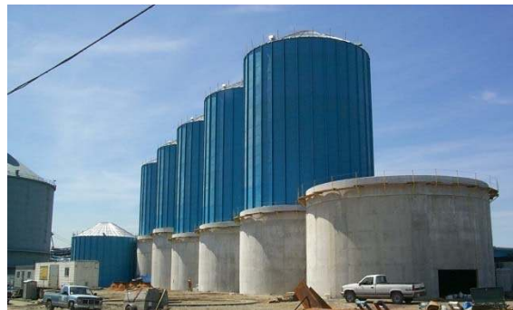
48' diameter silos under construction
