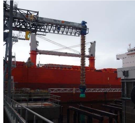
Figure 2.1-27 – Spout fully extended (Note depth below vessel deck)
