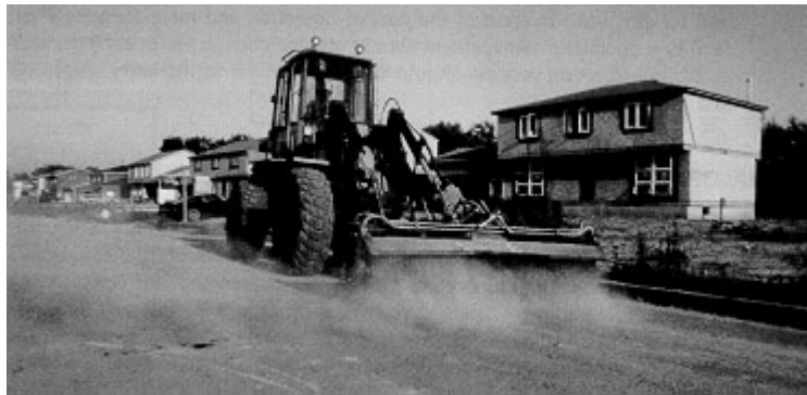
Figure 1-2: Residential Housing Construction (courtesy of Caterpillar, Inc.)
