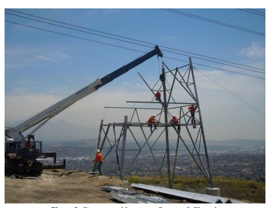
Figure 8: Crews assemble a tower, Segment 8, Phase 4.
