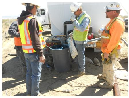
**Figure 2:** KV Structures mixing Revert Polymer with water at Tower M74-T1X, Segment 4.
