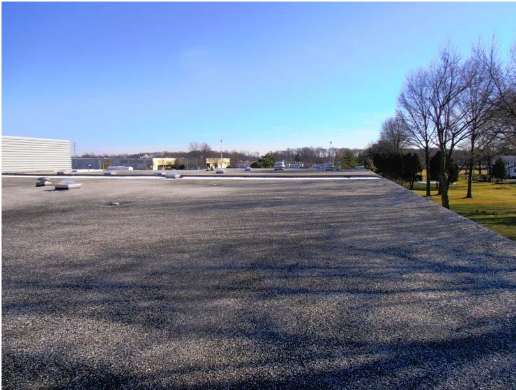
19. An additional overall photograph of Roof Area D.
