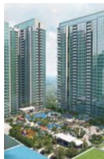
KOTA KASABLANKA Jakarta-Indonesia 202 Units Kitchen
