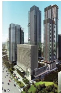
REGENT RESIDENCES Jakarta-Indonesia 113 Units Kitchen 170 Units Wardrobe
