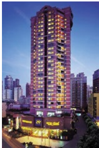
METROPARK Shanghai 187 Units Kitchen
