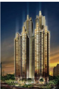
THE PEAK APARTMENT Jakarta-Indonesia 462 Units Kitchen
