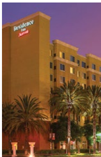
RESIDENCE INN ANAHEIM California US 108 Units Kitchen
