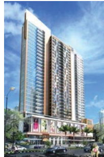
KEMANG MANSION Jakarta-Indonesia 312 Units Kitchen
