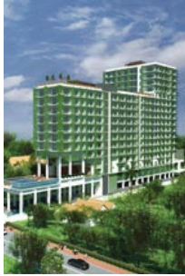
BELLEVUE SERVICED APARTMENT Cambodia 147 Units Kitchen 274 Units Wardrobe 243 Units Vanity 67 Units Laundry
