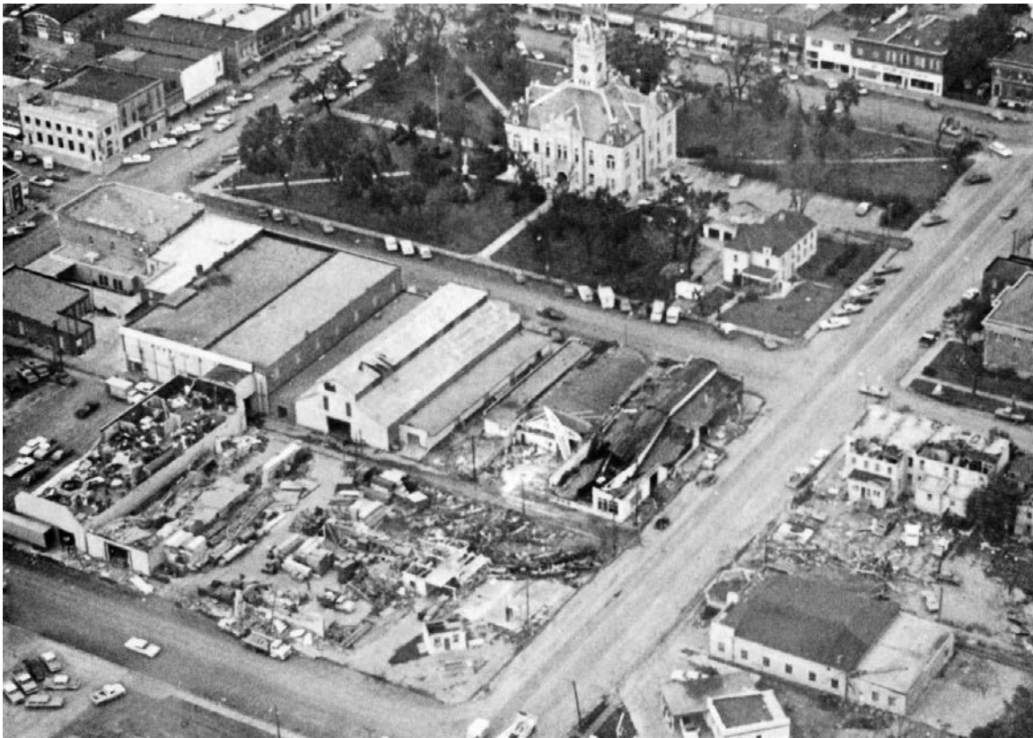
(Tornado damage, Dispatch pamphlet, September, 1973)
