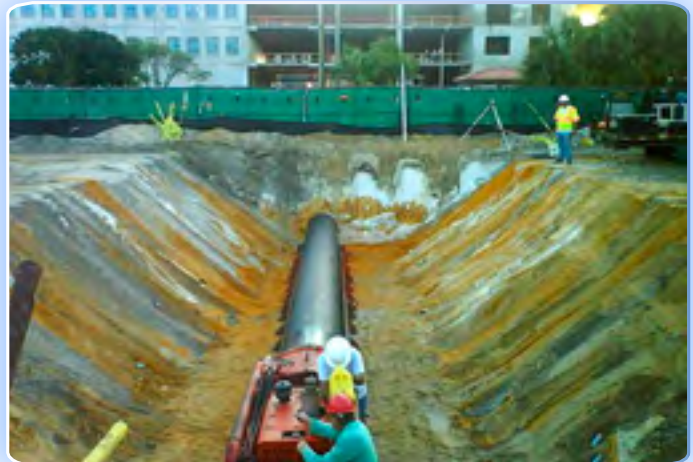
City Center West Palm Beach, FL Duct Bank System Around City Center In Downtown WPB Incorporating & Jack & Bore Across FEC Railway
