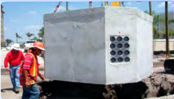
Lime Substation Interconnect Sarasota, FL Installed Duct Bank Infrastructure for the City of Sarasota included total 1000 KCMIL Copper Conductor installation in conjunction with an inter-city infrastructure upgrade & Loop Tie between substations.
