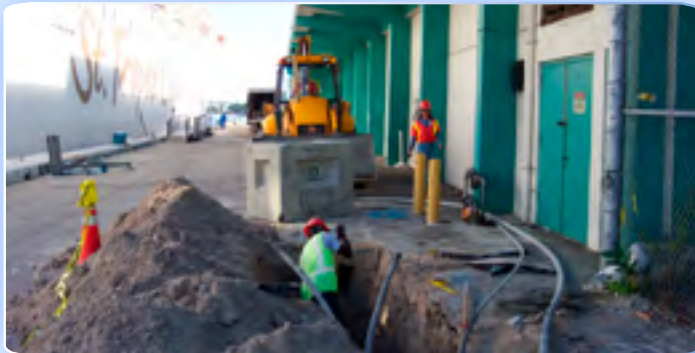
Terminal 18 at Port Everglades Fort Lauderdale, Florida Installation of 200+ Security Cameras, Conduit & Cat5 Cabling, Fiber Optic Cable, Network Switches & Nodes, Bridge Electrical Work
