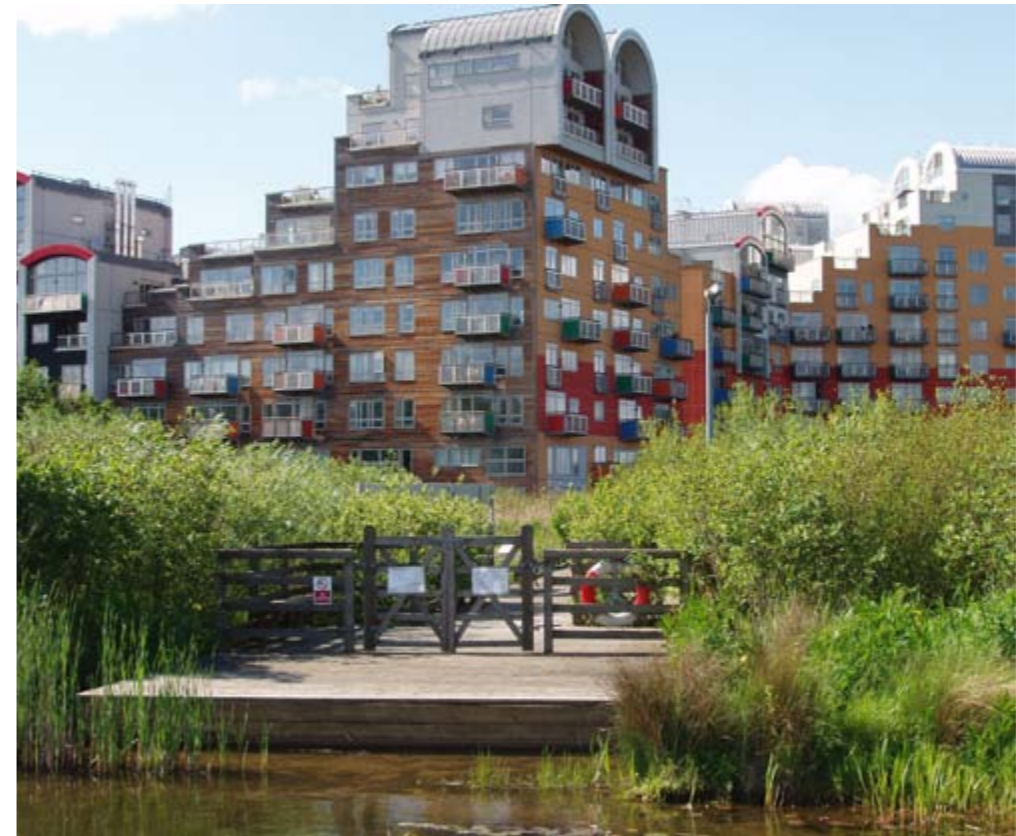
2. Examples of green infrastructure: ecology park at Greenwich Millennium Village.
