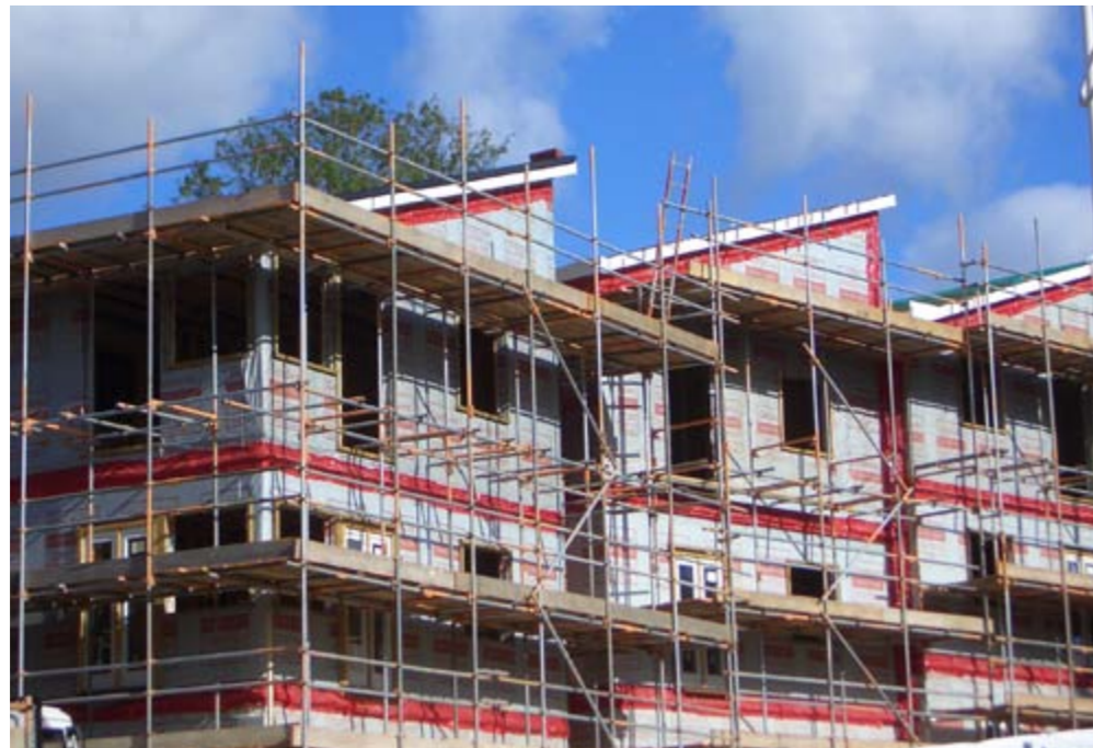
1. Operational development commenced following planning application approval.
