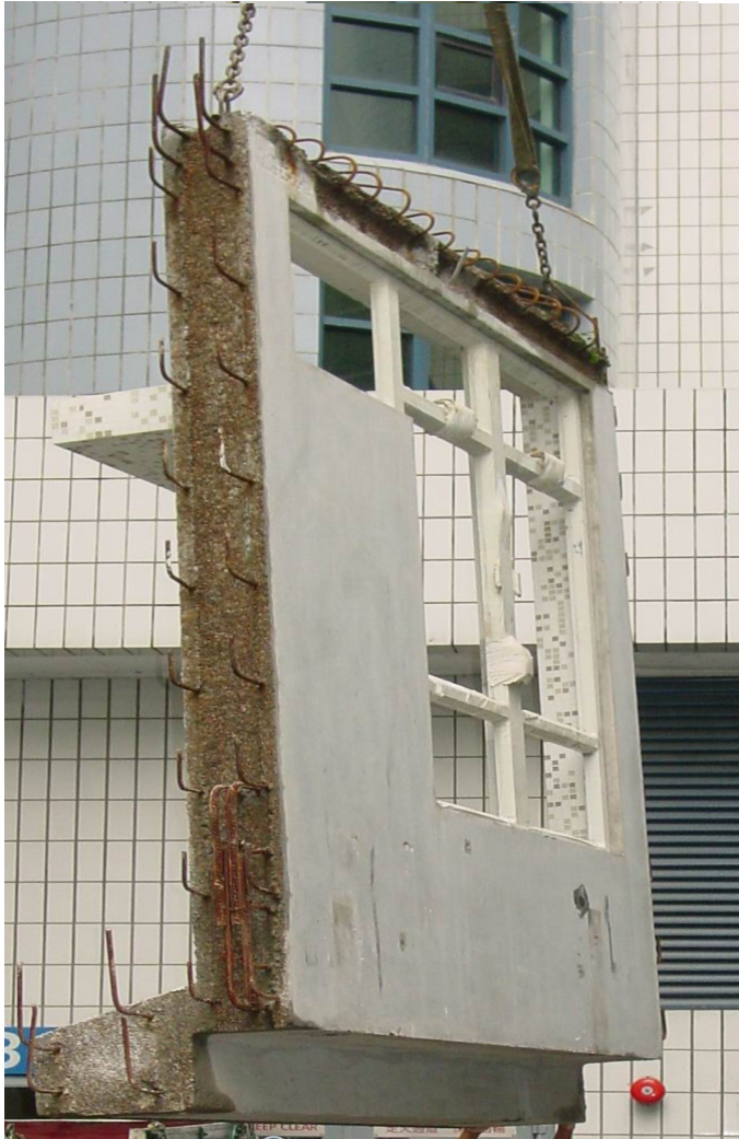
Fig. 3: Protocol of finished lightweight concrete precast façade
