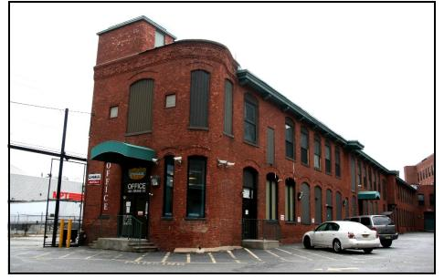
**BARBOUR 9:** oblique view looking SE of 1890 addition along Prince St. Note the rounded brick detailing in the cornice and lintels.
