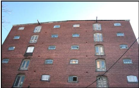
**BARBOUR 20:** detail view of north elevation, looking South from Grand St., showing hoisting beams and loading bays for each floor.
