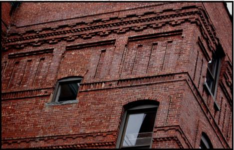
**BARBOUR 12:** close up view looking NW from interior courtyard. Note the extensive brick detail and corbelling in this view of the 1877 original building.
