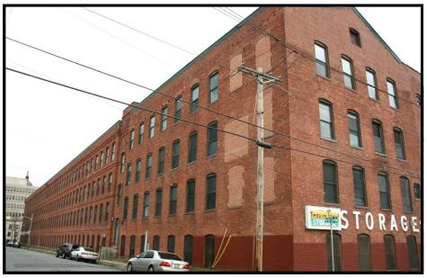
**BARBOUR14:** oblique view looking NE, showing Spring St. side. The joint between the 1877 building and the 1890 building is evident at left of center.
