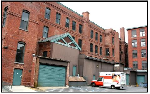
**BARBOUR 11:** oblique view looking NW into 1877 building. The rolling door and trestle area at center mark the location of the Boiler House that has been removed.
