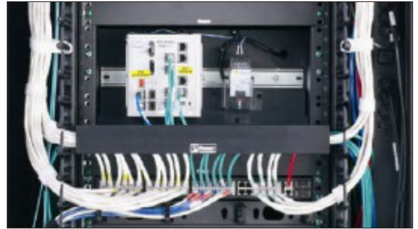
Figure 5. Manufacturing Switch Mounted on a DIN Rail Bracket
