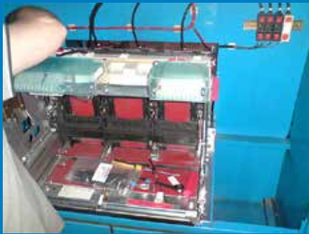
Direct Response Engineer Installing Retrofit ACB
