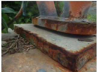
Corrosion on base plate and bearing plate File 085
