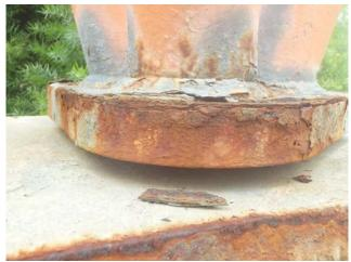
Corrosion on bearing plate File 087
