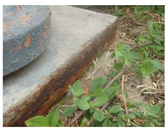
Corrosion on bearing plate File 089
