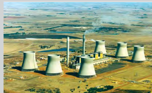
Indirect Dry Cooling South Africa
