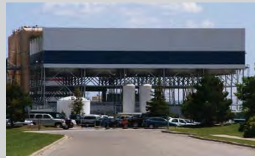
A-frame Air-cooled Condenser Canada
