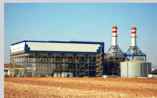
Air-cooled Condenser Spain
