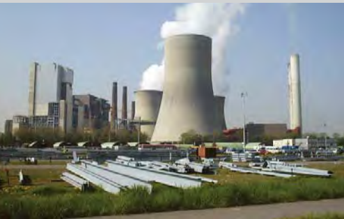
Natural Draft Cooling Tower Germany
