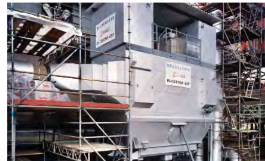
Bi-Corona® Electrostatic Precipitator
