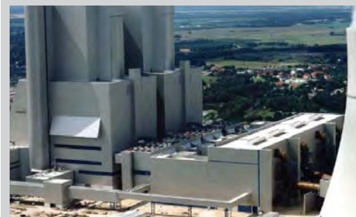
2 x 800 MW Air Preheater and ESP Project Germany
