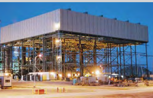
Air-cooled Condenser USA
