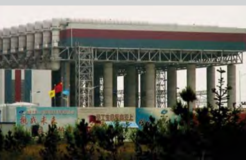
Air-cooled Condenser China
