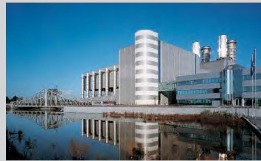
A-frame Air-cooled Condenser Belgium
