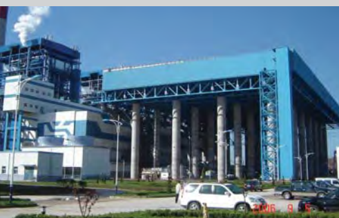
Air-cooled Condenser China
